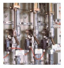
With more or less pressure The carbon dioxide is supplied in high-pressure cylinders or low-pressure vessels. The optimum supply method depends on the quantity of extinguishant required and the particular circumstances.
